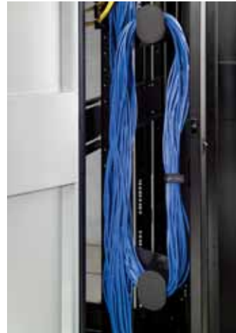
Vertical cable management channel
